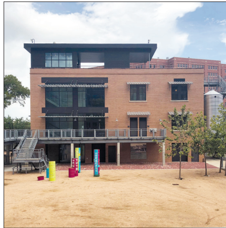
Fig. 5. Sunset Coffee Building, along the Buffalo Bayou, Houston, Texas, built 1910, photograph 2018. The building had been recently renovated when Hurricane Harvey hit in 2017. While the rehabilitation was designed to withstand flooding, the building did sustain damage to its elevators and electrical systems. Courtesy of Priya Jain.
