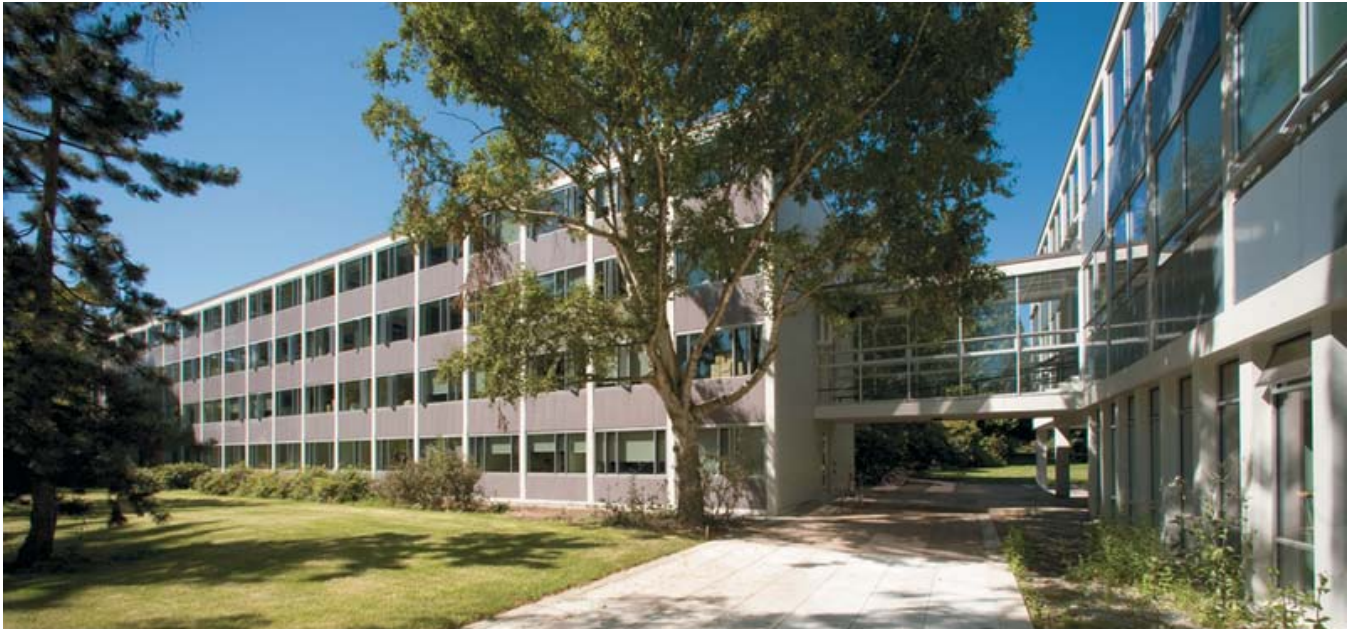
REHABILITATED MODERN EXTERIOR ENVELOPE ASSEMBLY. BUCHANAN COMPLEX, UBC. IMAGE: PERKINS + WILL
