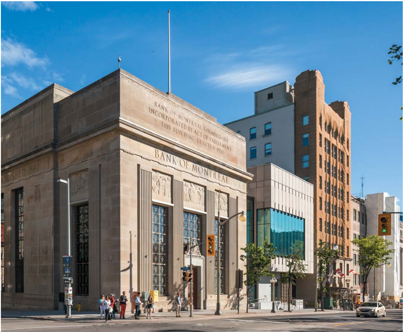
IR JOHN A. MACDONALD BUILDING REHABILITATION ADDITION AND ADAPTIVE REUSE, OTTAWA. WELLINGTON STREET VIEW ACROSS FROM PARLIAMENT BUILDINGS; REHABILITATION OF THE ORIGINAL 1932 BANK IS COMPLETE; CONSTRUCTION OF THE NEW ADDITION IS ALMOST COMPLETE IN THIS PHOTO. THE PROJECT IS ON TARGET TO ATTAIN A GREEN GLOBES® 70 SUSTAINABILITY RATING (EQUIVALENT TO LEED SILVER). ARCHITECTS: NORR/MTBA PHOTO: DOUBLESPEACE
