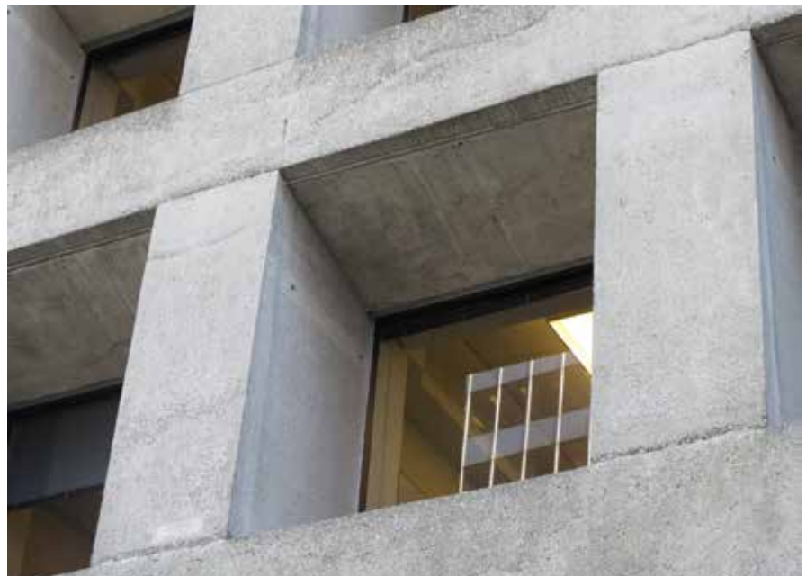
Poured-in-place exterior concrete facade. MacMillan Bloedel Building. Vancouver, BC. MTBA Inc.
