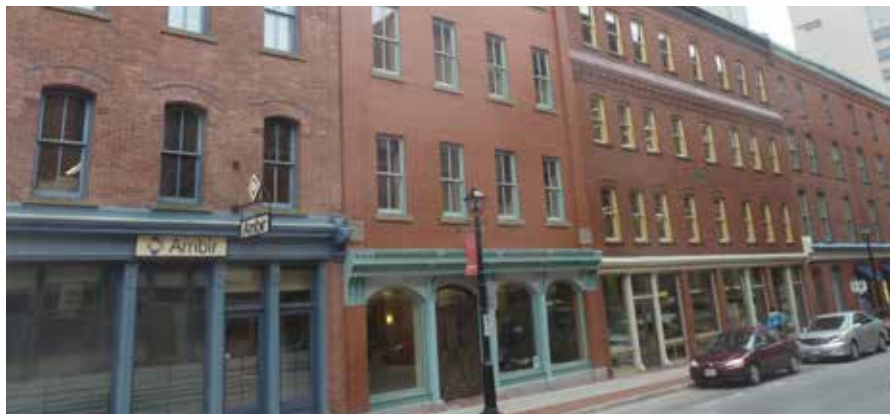
New Construction (infill) fills former void in streetscape and is designed sensitively in context using compatibly sized windows and materials. Jim Bezanson.
