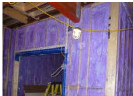
Clockwise from top left: Diagram illustrates "box within a box" approach; Detail of exterior brick cladding; Vent detail at south wall double window cavity; Construction image showing insulation of interior wall assembly; The house prior to rehabilitation. ERA Architects.
