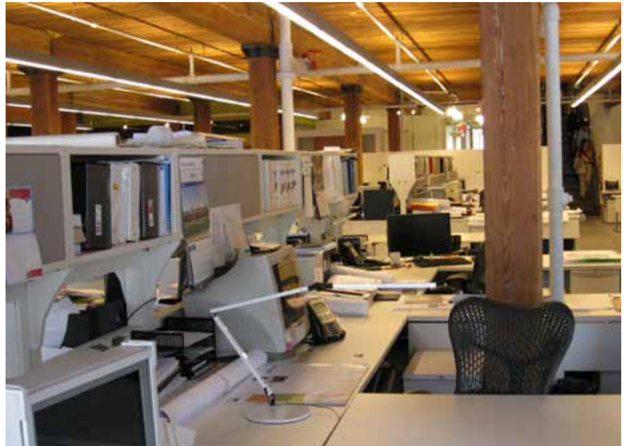
Task lighting with personal control. Former McGregor Sock Factory (Stantec Offices) Toronto, ON. MTBA Inc.
