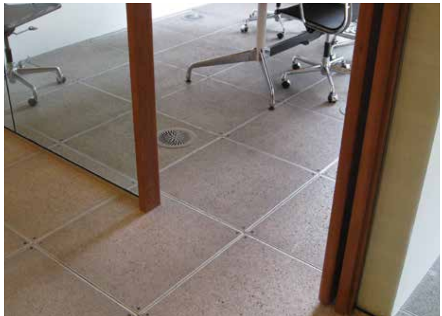
Raised floor system installed in historic building. Former McGregor Sock Factory (now Stantec Offices), Toronto, ON. MTBA Inc.
