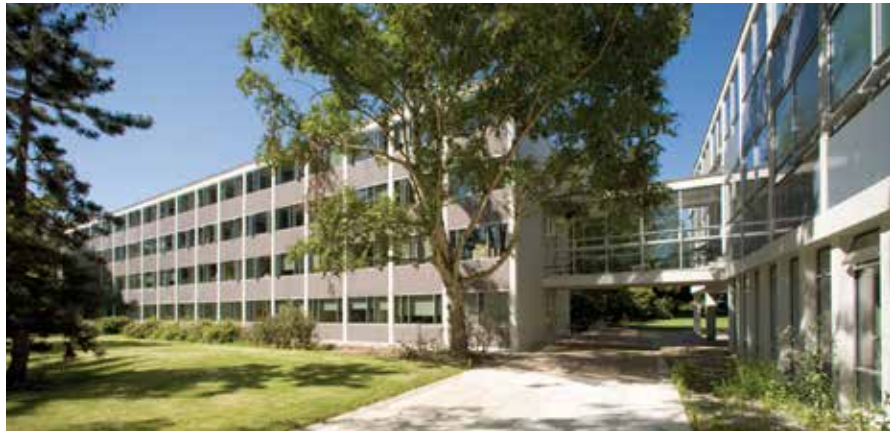
Rehabilitated exterior assembly. Friedman Building, University of British Columbia Acton Ostry
