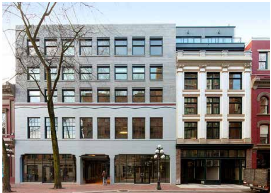
Rehabilitated storefronts with transoms. The taller storefront glazing provides light deeper into the ground floor storefront. Vancouver, BC. Acton Ostry.
