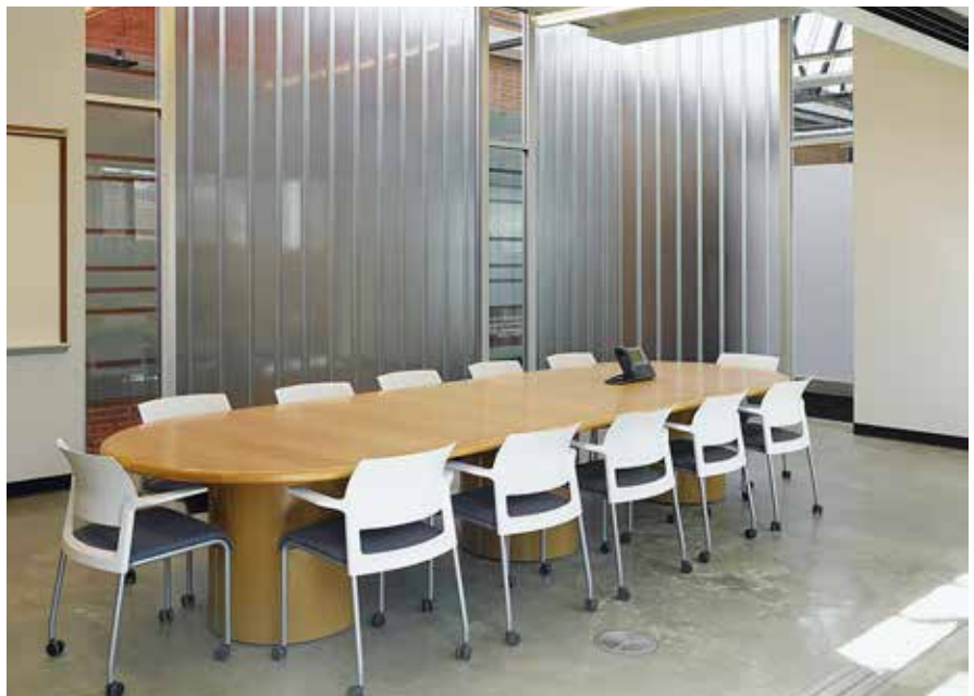
New glazed partitions used to enclose meeting room, allowing natural light to penetrate into room from central skylit space. Triffo Hall. Barry Johns Architecture Limited.
