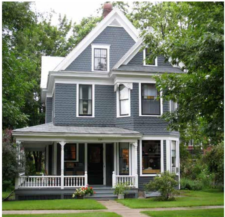
Front porches on early single-family residences such as this one in Fredericton, NB provide both shade and an opportunity for natural cross ventilation. Shelley Bruce.
