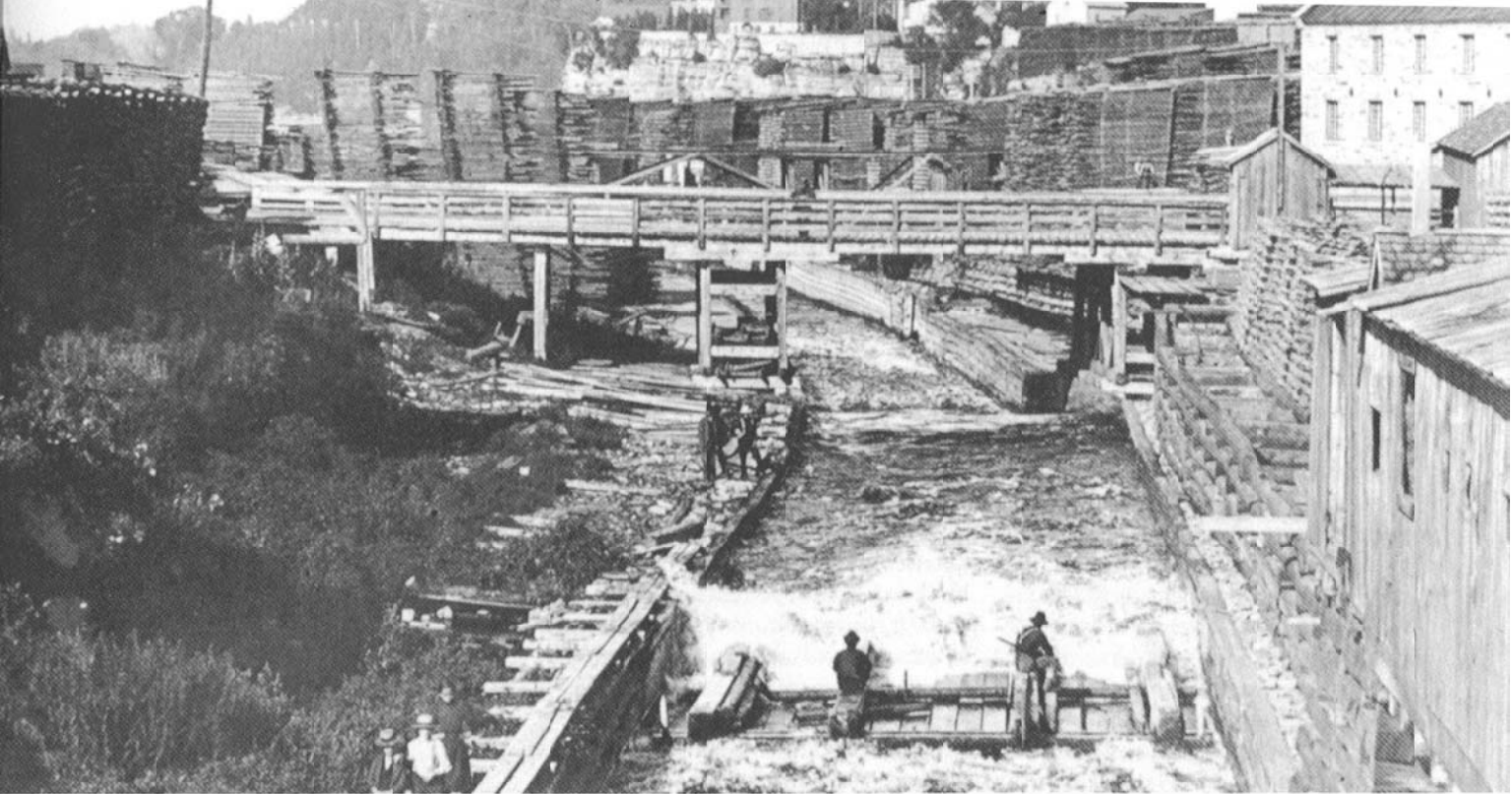
Timber slide at Chaudière Falls, c. 1890. Photo: National Archives of Canada
